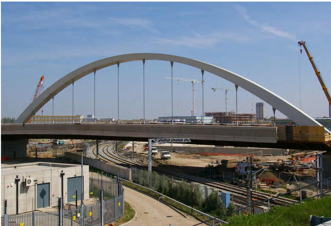
Figure 9: Example Tied Arch Bridge
